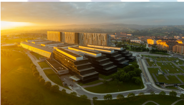
Central University Hospital of Asturias, Oviedo, Spain
